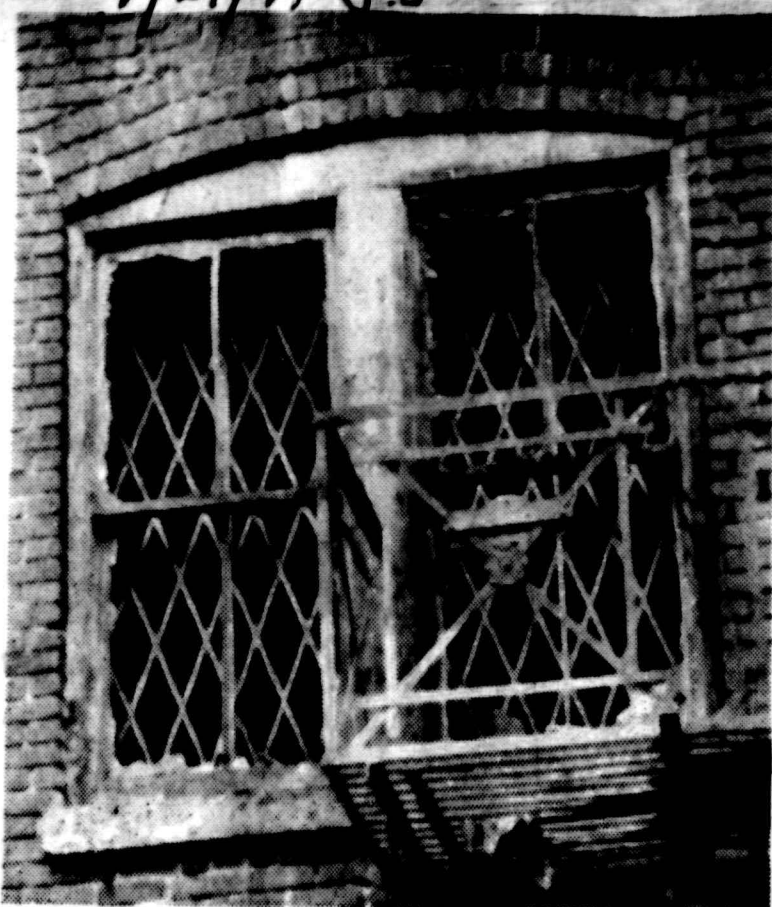
These metal grates on the windows of one of the fire ravaged buildings on Clinton Street in Hoboken are prevalent but illegal throughout Hudson County because they make escape or rescue almost impossible.
