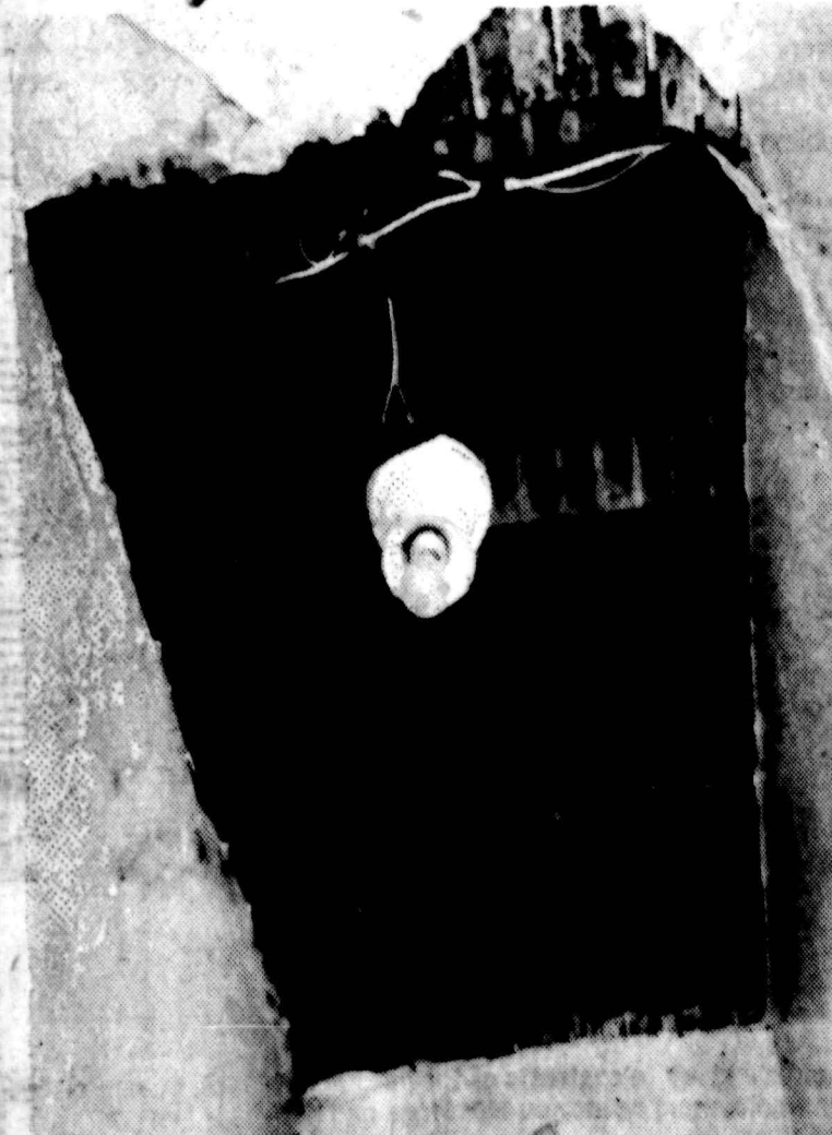
Among the building code violations at 527 Willow Ave. in Hoboken are these exposed electrical wires in a bathroom.
