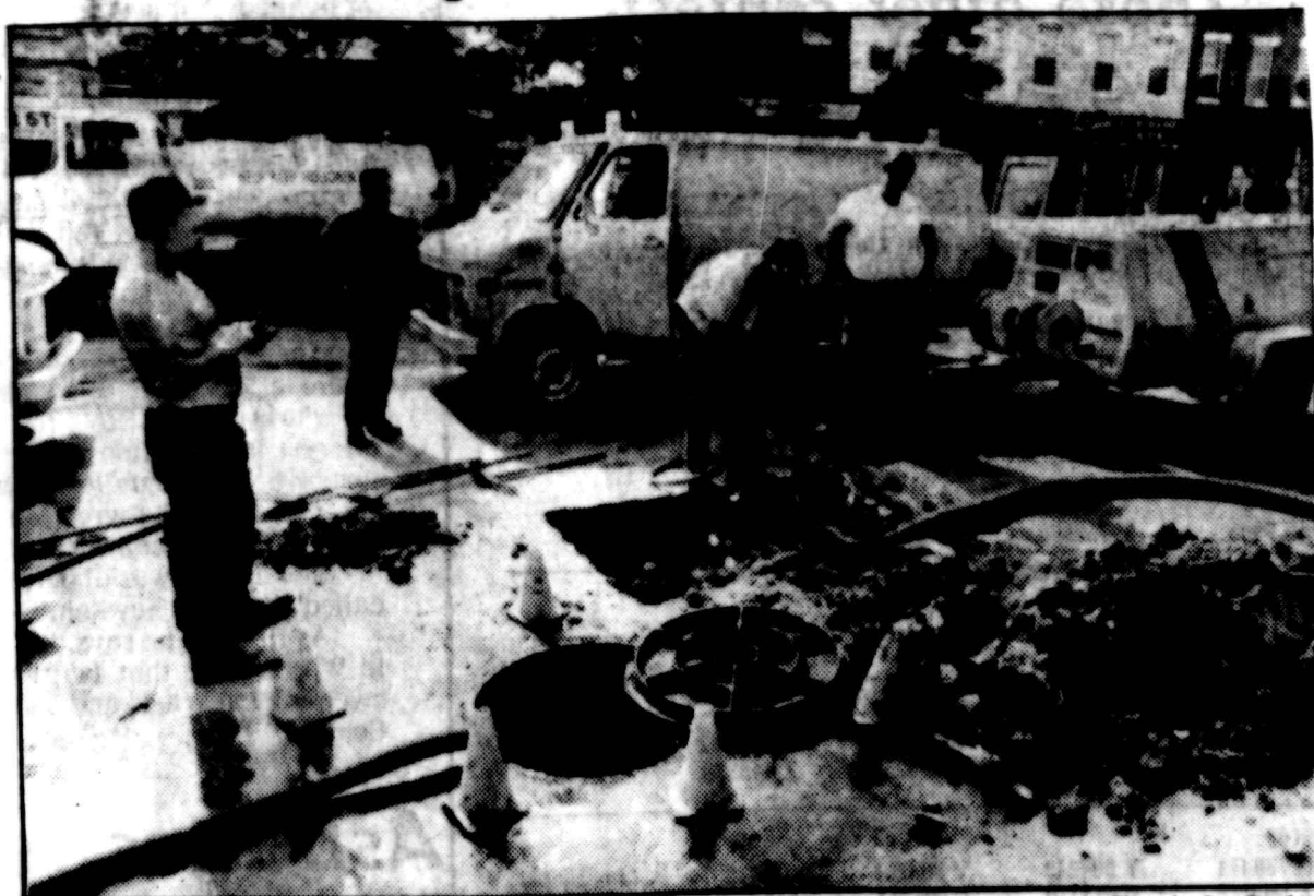
Hoboken Public Works employees repair a broken water main under Washington Street. It left many residents without water and snarled traffic yesterday.
