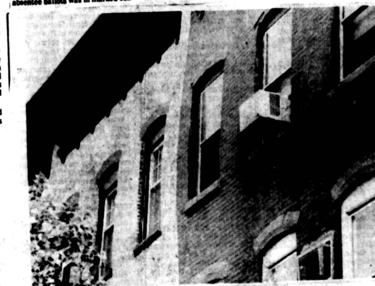
These facades at 417-419 Washington St. in Hoboken appear to be buckling outward and in danger of collapsing yesterday.
