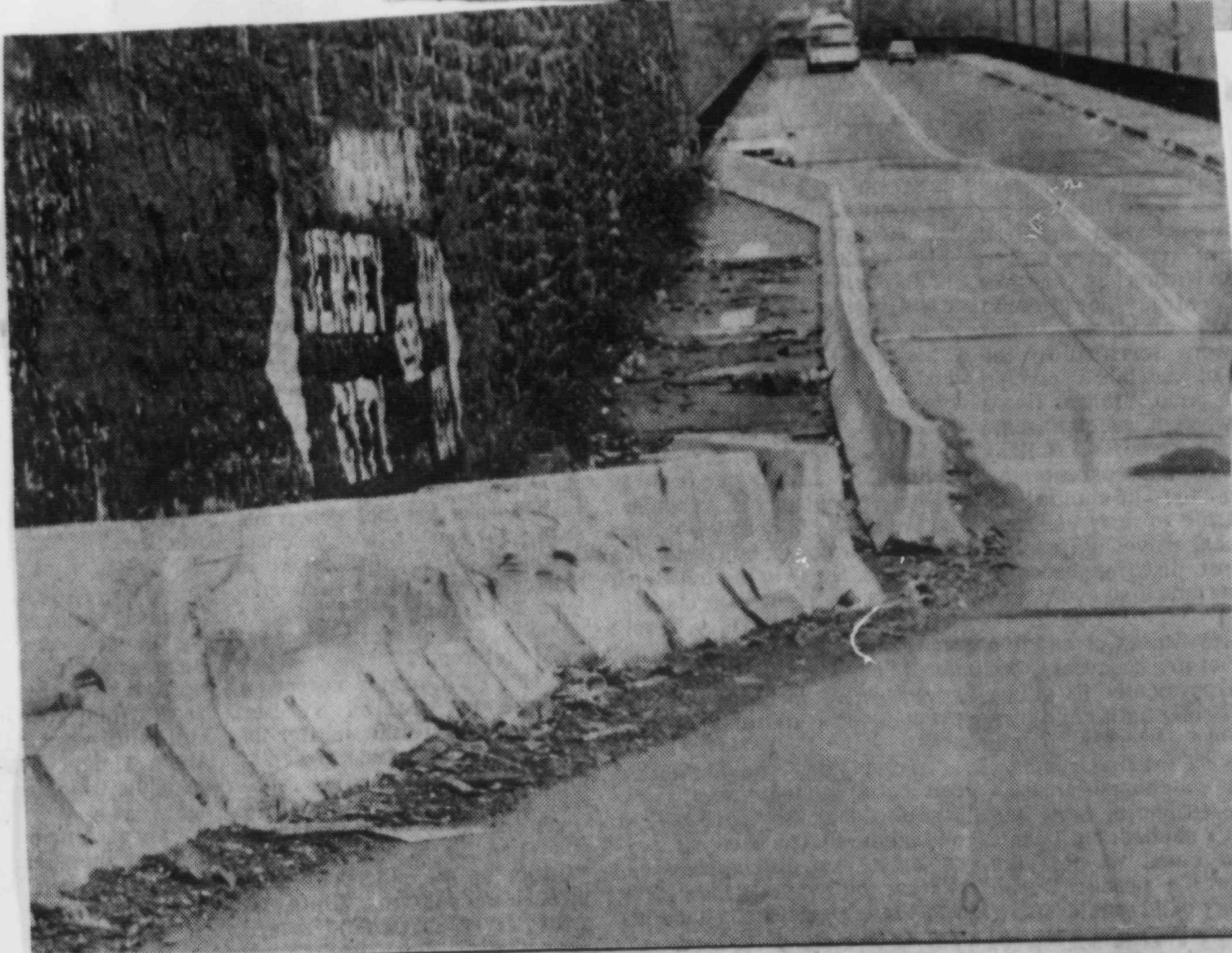
BATTERED ABUTMENT —A concrete abutment along the south wing of the viaduct leading into Jersey City bears the marks of many collisions with passing automobiles. Hudson County police reported six accidents due to the abutment in one 12-week period.
