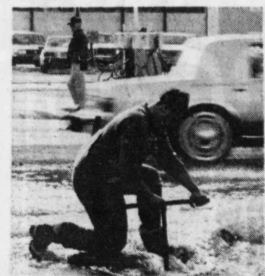
A Public Works Department employee slowly closes the valve, photo left, to reveal the cracked and broken pavement above the leak.
