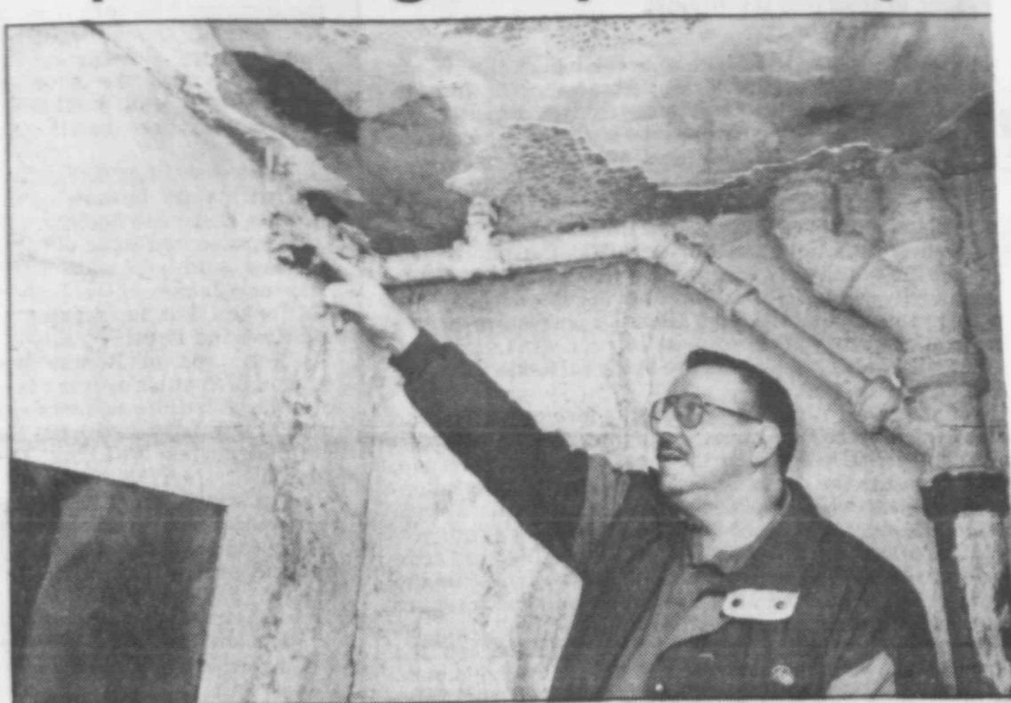
Frank Mannino, a member of a social club that meets at 504 4th St., Hoboken, points out crumbling ceiling caused by leaking water pipes.
