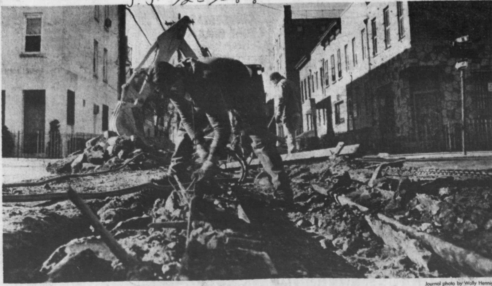
Workman Ron Paige cuts through old trolley tracks during construction on Second Street, Hoboken.
