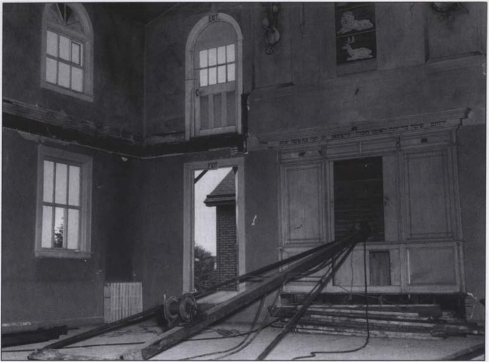
BLANCHE STREET SYNAGOGUE. By 1952, the synagogue was getting older. It then became home to the Linden Police Athletic League. This scene shows the interior of the synagogue as it was being transformed to hold a gymnasium for the PAL. (Courtesy Maureen Edwards.)
