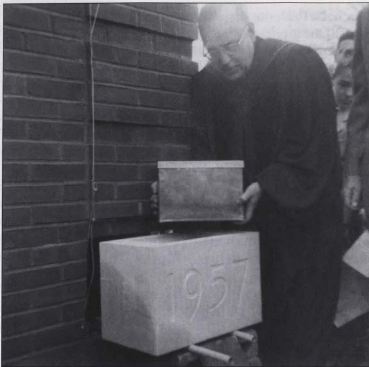
REVEREND KENNETH WALTER. The reverend is setting the cornerstone of the Linden Presbyterian Church's addition of the church school in 1957.
