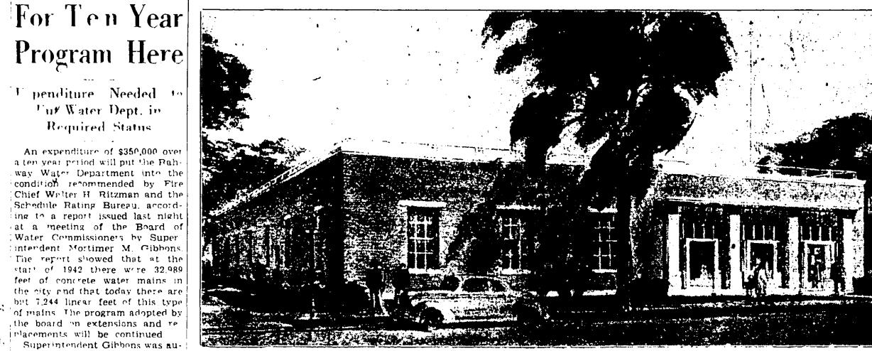
Above is the architect's sketch of new telephone building to be built on West Milton avenue brick construction, frontage is 90 feet with 127 foot depth along Georgia street.
