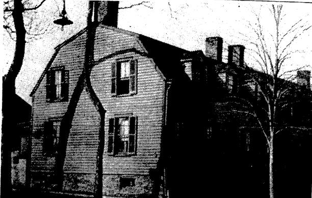
NO LONGER AROUND - The old Marsh homestead in dows, was built in 1730. Its chimneys are typical of the lation of the support we sion 222. Rahway was located at the junction of Elm Ave. and Georgian period and the foundation was constructed have received from thou-West Main St. The colonial structure, with a gambrel from fieldstone. This picture was taken from one of the sands of Americans for our
