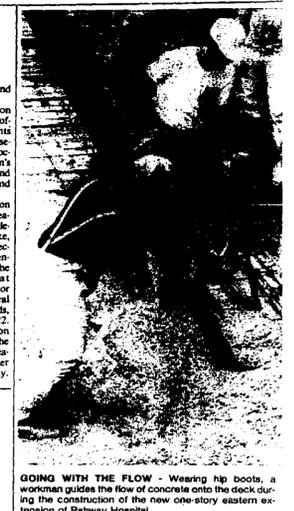
GOING WITH THE FLOW - Working NP boots, a worker guides the flow of concrete onto the steel structure of the new one-story extension of Rahway Hospital.
