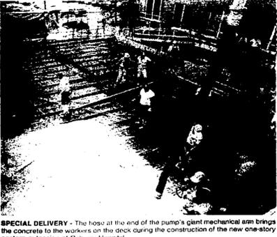
SPECIAL DELIVERY - The hose at the end of the pump's giant mechanical arm brings the concrete to the workers on the deck during the construction of the new one-story eastern extension of Rahway Hospital.
