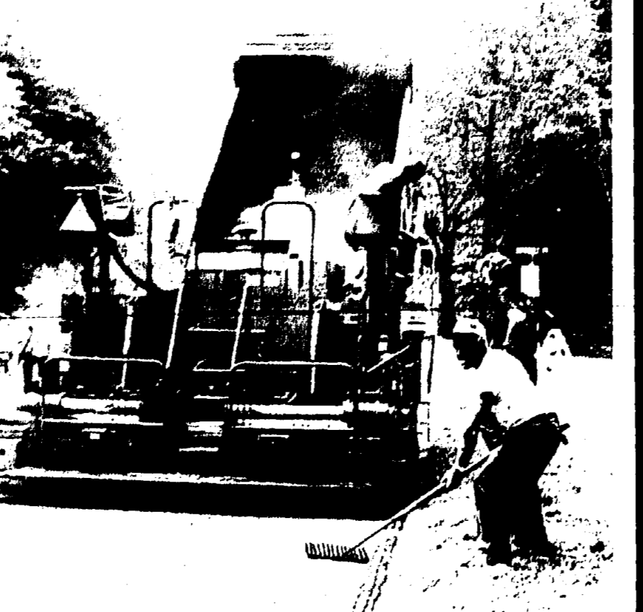
RESURFACING UNDERWAY... The Super 8s of the Union County Department of Public Works recently finished resurfacing and repaving a three-quarter mile stretch of Gullwing Hill Rd.
