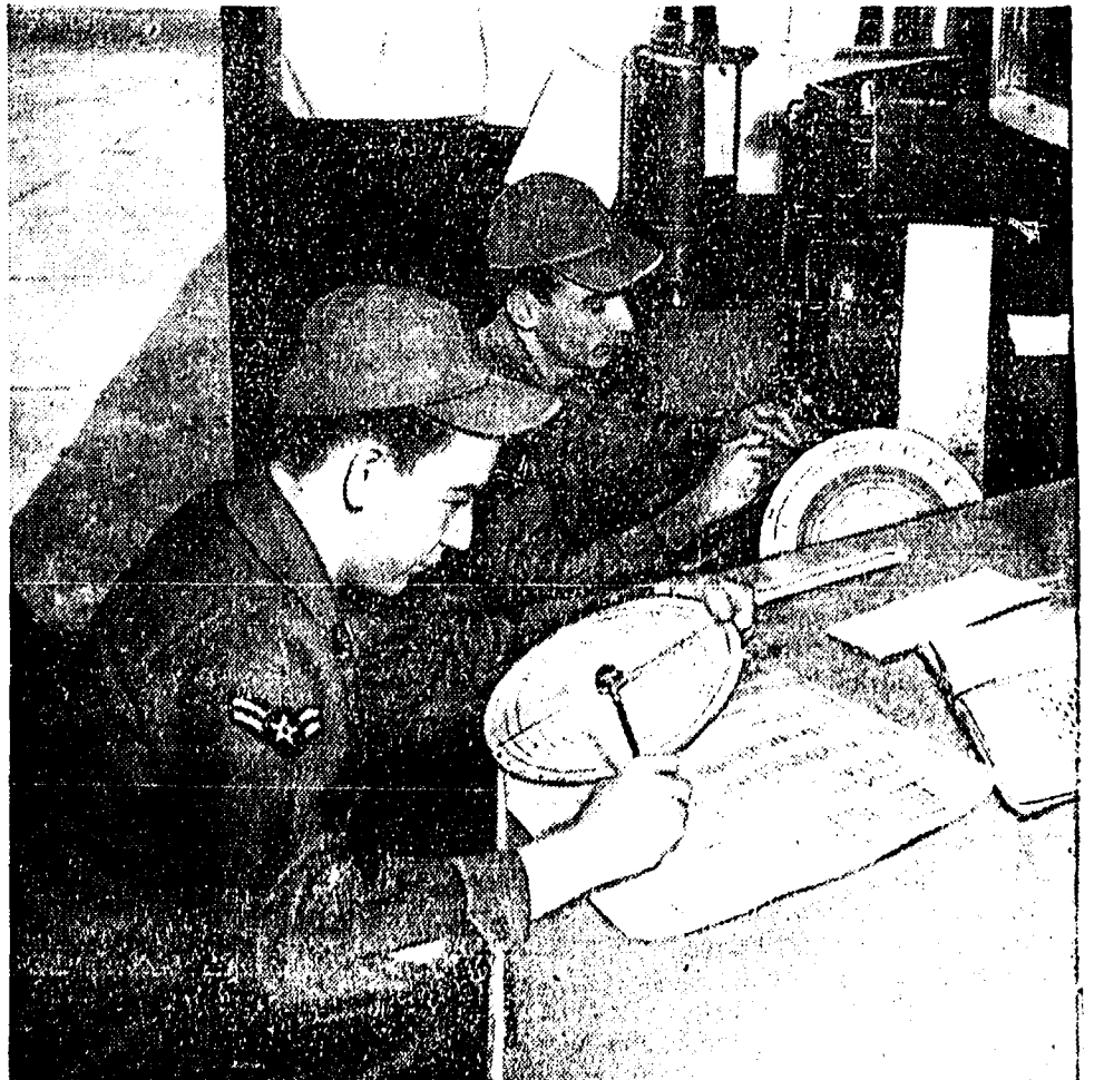
Airman Charles Mills threads tape recorder to read back data sent to it by the tiny radio aloft. Airman John Willis prepares to log the information.
