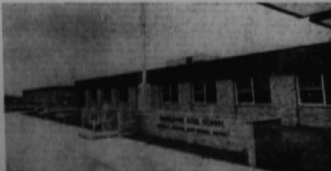
ONE OF FIVE — Manalapan High School is one of five high schools in the Freehold Regional High School district which serves eight municipalities in western Monmouth. There has been increased
