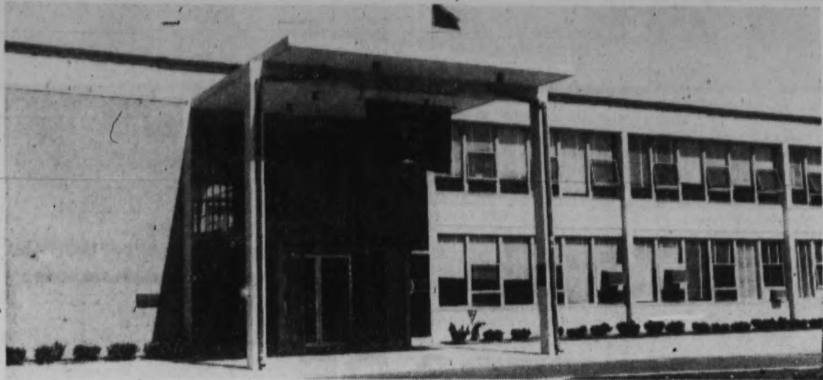
HALL AND FAREWELL—Myer Hall, above, is the headquarters of the 11-building complex the Army Signal School is vacating at Ft. Monmouth. The Army has confirmed that it won't
