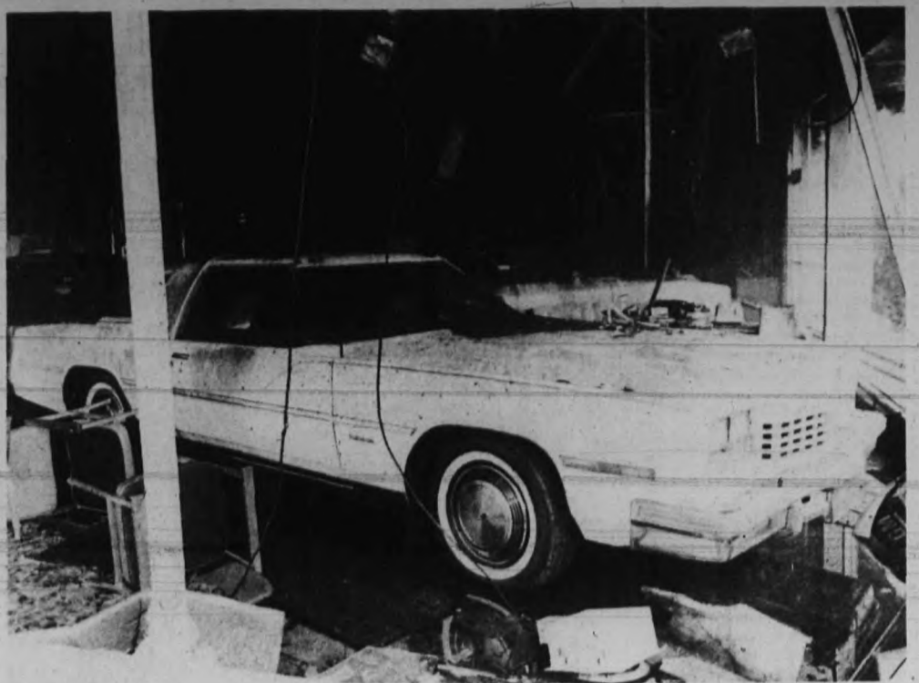
DAMAGED CARS — Six new cars in the showroom and about a dozen in the garage of the car dealership were damaged by the fire. An early report by Keyport police said faulty electrical wiring appeared to be the cause of the blaze, and Fire Chief
