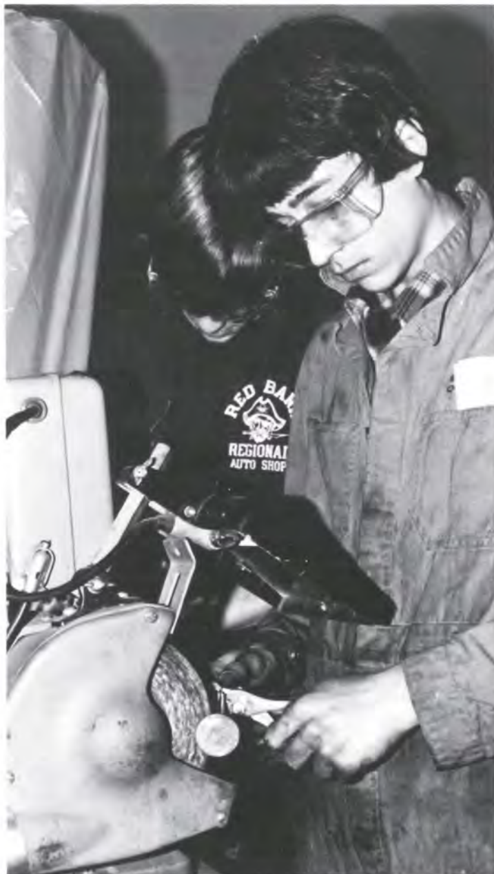
Chad Heulitt watches Drew Sciculino clean the carbon off a valve.
