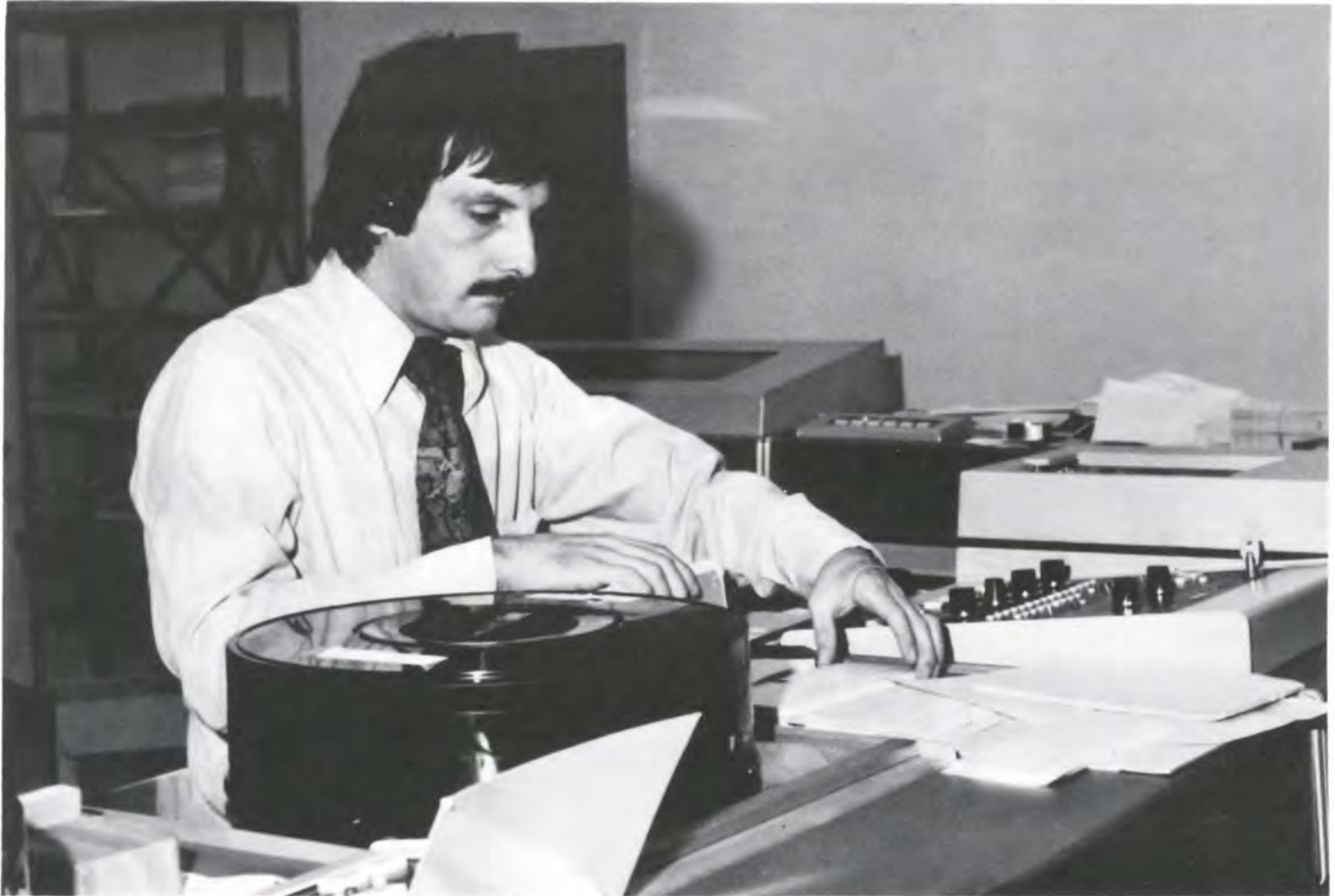
Mr. John Galloway loads a program into the computer. The cards tell which program to access for memory.
