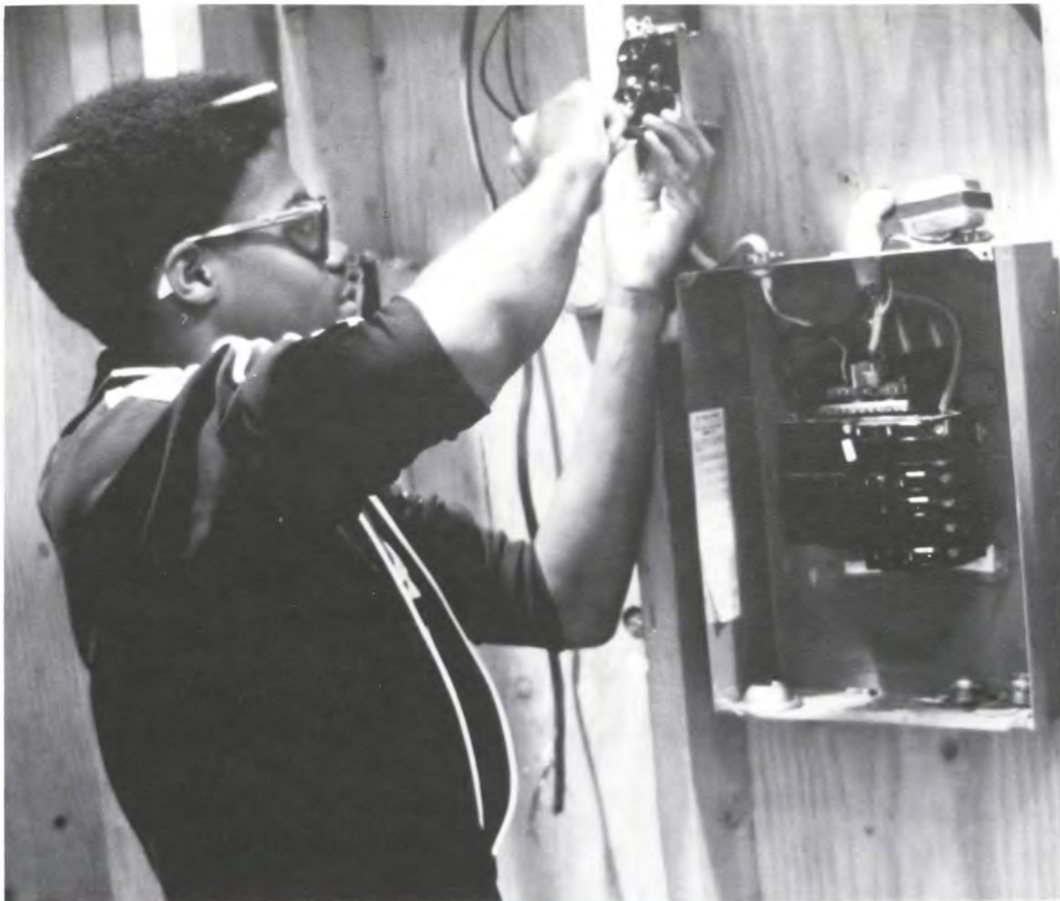
Sam Jones installs a duplex outlet inside the storage shed built by Mr. Warren Booth's Building Trades students.
