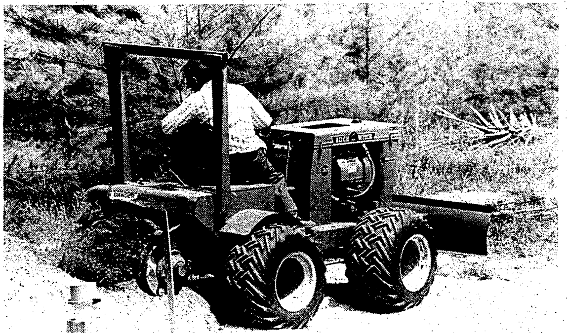
Powerful 'Ditch Witch' tractor churns dirt prior to installation of an underground telephone cable at Mariner Pointe condominiums. Mariner Properties, the developer of the Causeway Road project, received the go ahead Tuesday to complete 16 of the 25 units planned in the final phase of the development.
