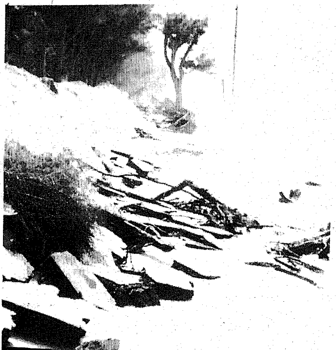
Same road, same time, beach side view. Those chunks you see used to be a road quite a few feet higher.
