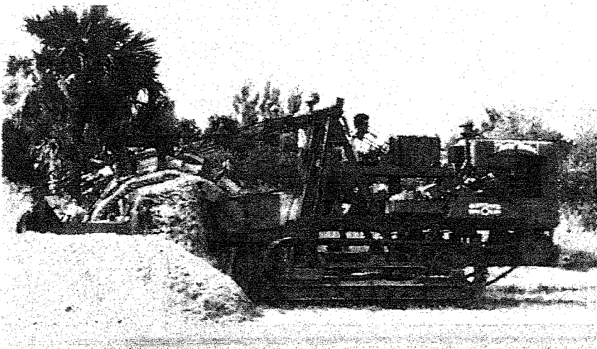
Installing water mains on Sanibel Island
