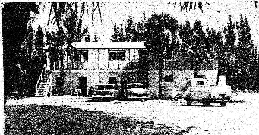
Golden Shell Apartments Near Completion
