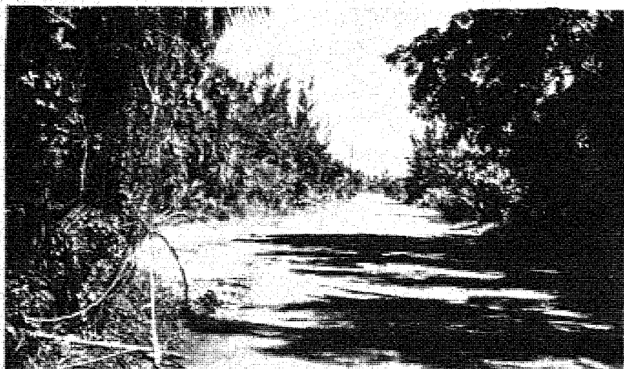
Tulipa Way is now paved
