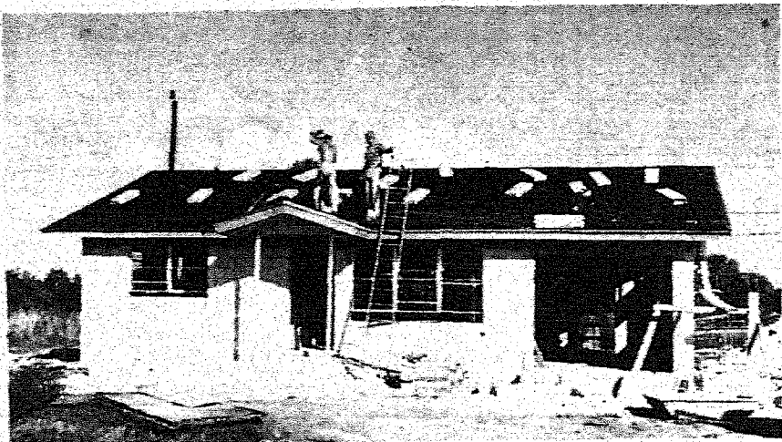
NEW HOME CONSTRUCTION IN TRADEWINDS
