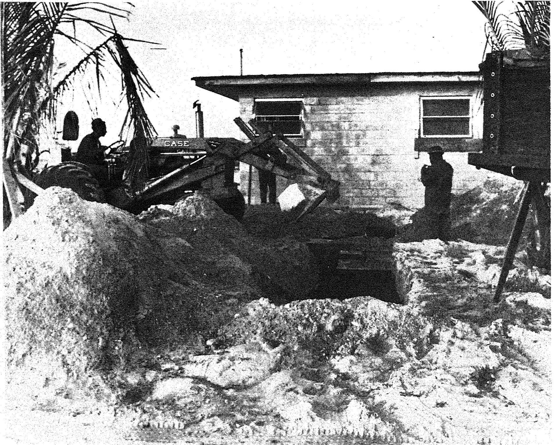
COUNTY WORKERS AT WORK ON THE REST ROOM FACILITIES ON THE CAUSEWAY.
