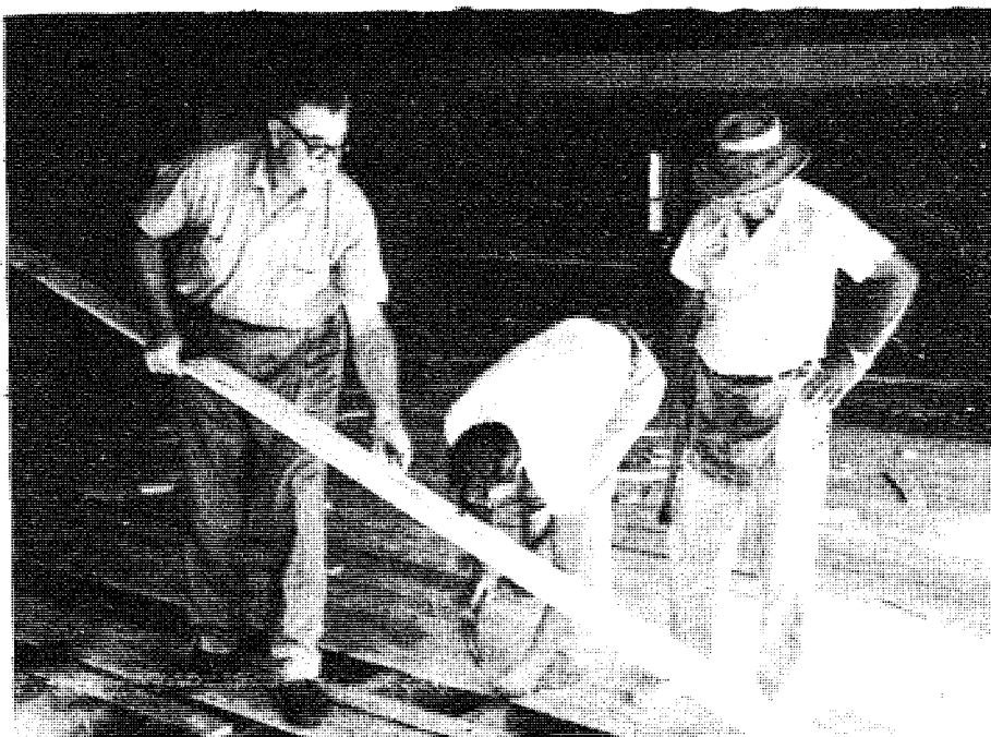
Laying flooring in the new addition are from left to right, Gerry Martin, Tom Nix and Floyd Pflough.
