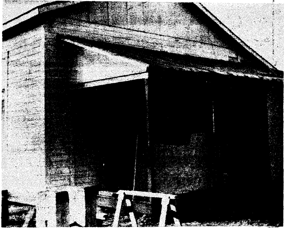
Here's the way the old Sanibel Schoolhouse looked when the Hunters bought it. That's Ralph Woodring on the front porch, little realizing when he attended the Island schoolhouse as a boy, he would one day be wielding a hammer to make it the Islands' Pirate Playhouse.
