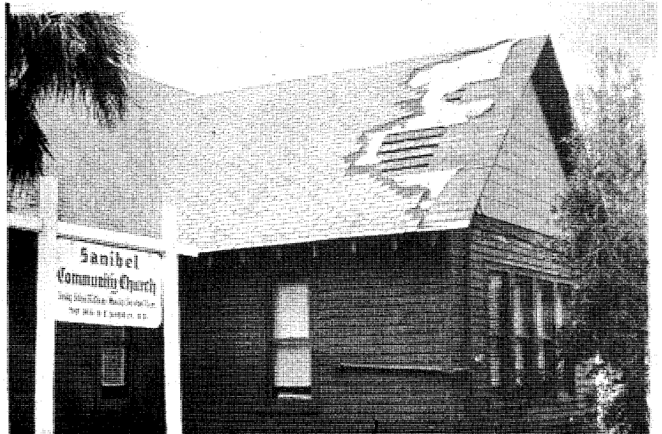
The damage to the roof of Sanibel's oldest church, The Sanibel Community Church, located directly in back of the demolished Town Square.
