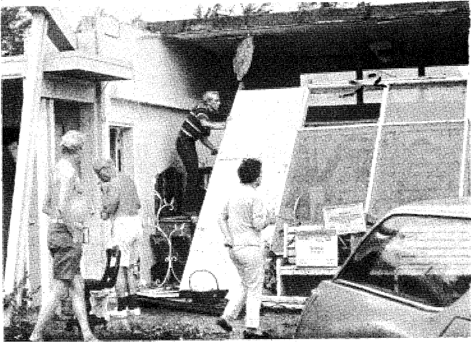
The remains of Serendipity Antiques --- at least a couple of feet of roof remains, although not for any obvious purpose, we guess.
