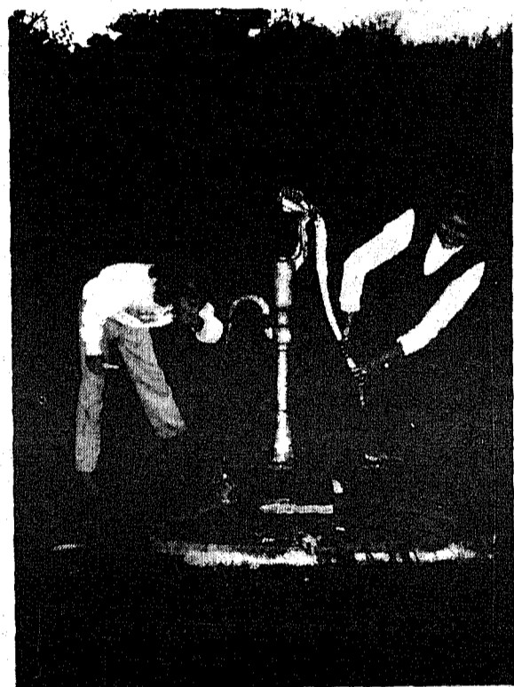
where even city gals can use a pump
