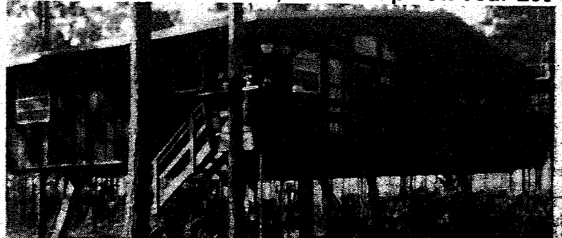
SOLID STEEL FRAME, RESTING EIGHT FEET ABOVE THE EARTH, ANCHORED IN RE-INFORCED CONCRETE FOOTERS LOCATED BENEATH THE SURFACE. CORNER STANCHIONS BRACE IN TWO DIRECTIONS.
