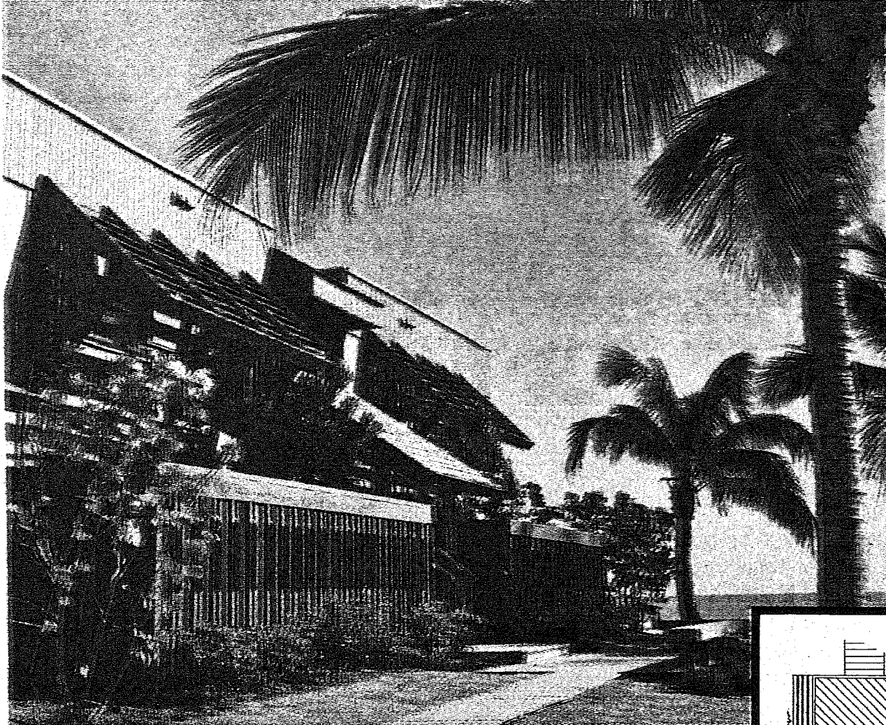
The white stuff just beyond the front door of the first building at Sanibel Beach Club is not snow.
