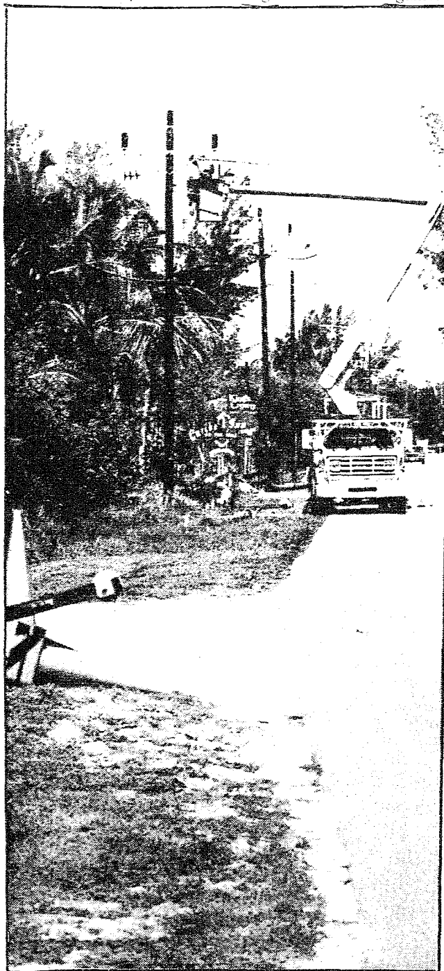
Traffic has been slowed on West Gulf Drive crews from Koehler Construction installed new power poles.
