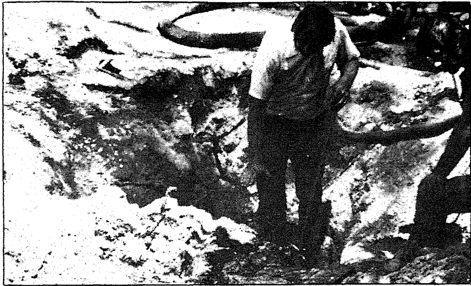
The sinking situation on the bike path has been resolved with concrete pipe and hard work.
