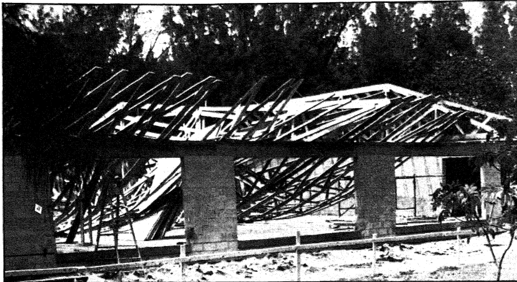
These roof trusses on the new building at Periwinkle Place came crashing down like a row of dominoes Friday afternoon when plywood was stacked on them. Dame Fortune was smiling though and no one was hurt.
