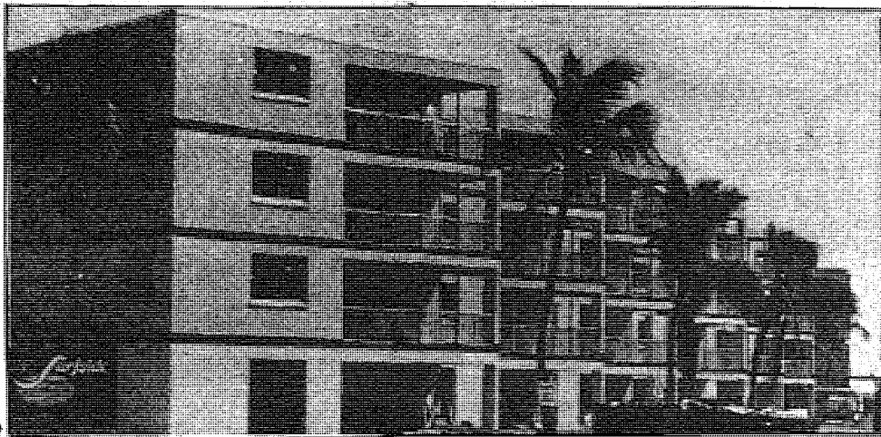
Sanibel Surfside, a 30-unit condominium on the Gulf, rapidly nears completion.
