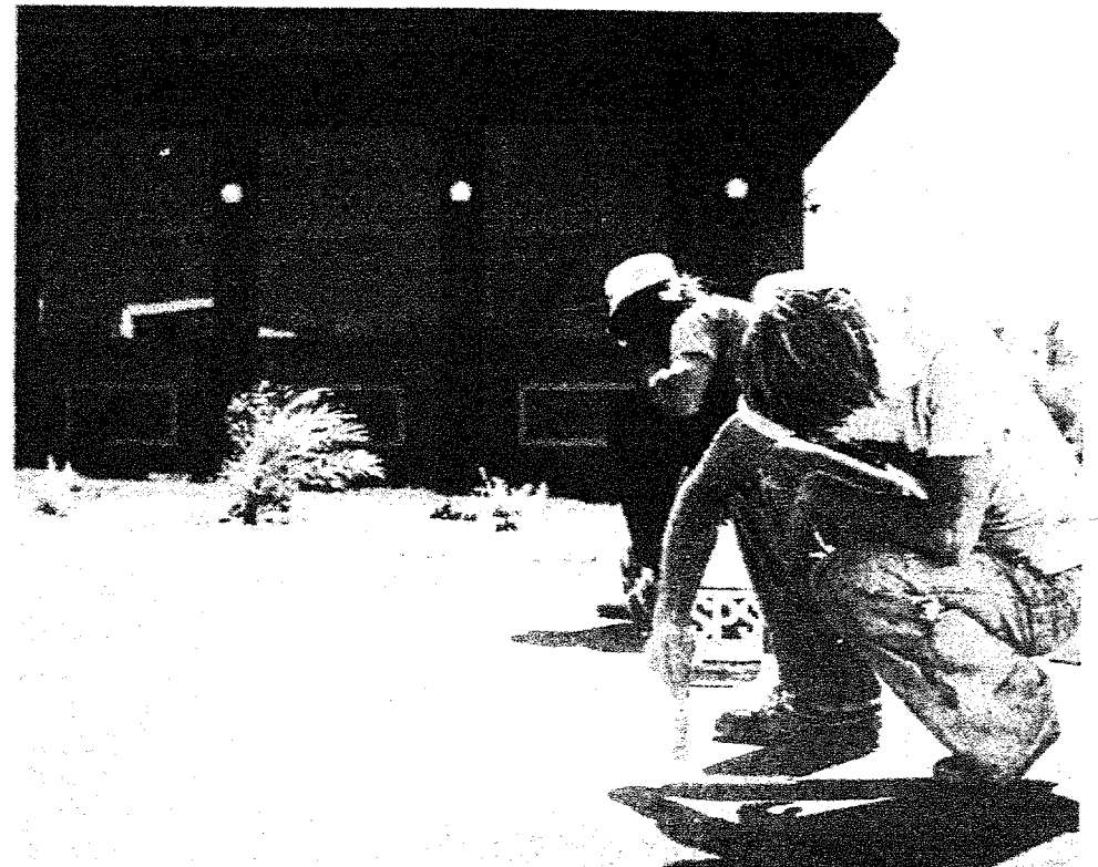
Regency employees apply a surfacing to a parking lot.
