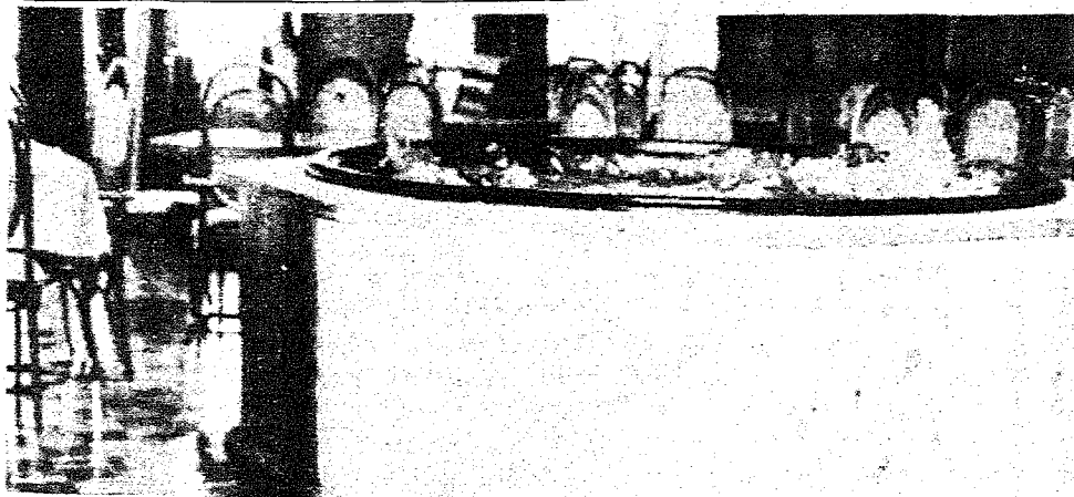
The interior construction is almost finished at Chez Rondolet, the new restaurant in the round at Tahitian Gardens. The 250-plus seat restaurant will feature a fountain in the center of the new eaterie. Estimates on the exact opening date were not available at press time.
