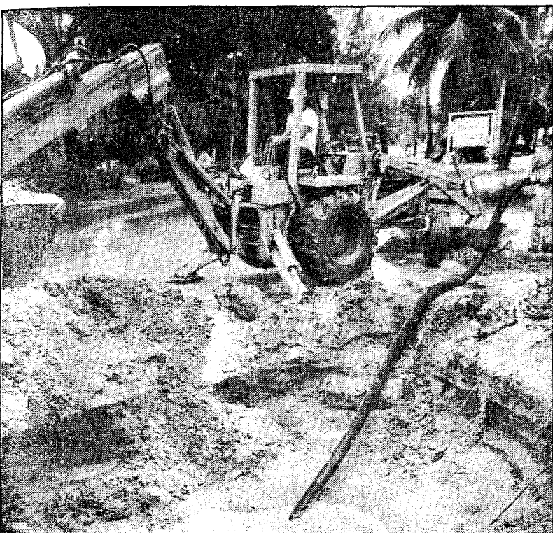
Bob McDaniel throws the broken water line coupler out of the service hole in front of the Bait Box. The tree root in the bottom right hand corner was the culprit that broke the coupler.
