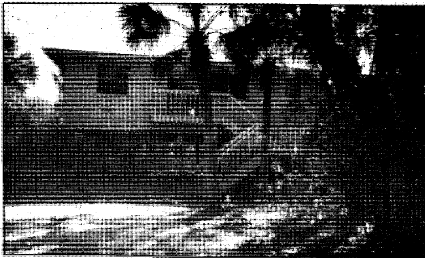
CAPTIVA private setting for this 3 bedroom; 2 bath home. Wood frame on piling new home. Large screened lanai. Pleasingly furnished with wicker and earthtone colors throughout. This carefree home is ready for occupancy and requires nothing more than you and your luggage. Call us for financing terms and appointment to see this charming place.
