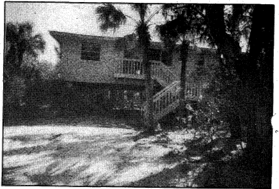
Captiva privacy can be enjoyed in this three bedroom, two bath, wood frame piling home with large screened lanai. Pleasingly furnished with wicker for a Floridian decor. This carefree home is ready for occupancy and offered completely furnished at $225,000 or, if you prefer, unfurnished, at $200,000. Financing terms are available.
