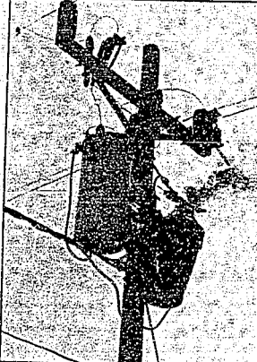
Power was knocked out temporarily last Wednesday when this transformer exploded near the Beachview Country Club. Photo by Mark Johnson.
