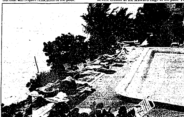
The pool at Ocean's Reach condominiums must be moved if the rock revetment is constructed.
