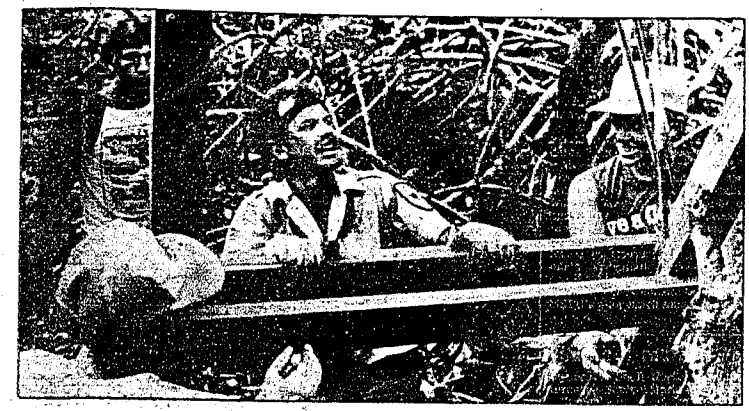
Supervisor Richard Blackburn works alongside Brian Willis, Peter Butler and Steve Martin setting up a support for the continuation of the Gasparilla Trail boardwalk.
