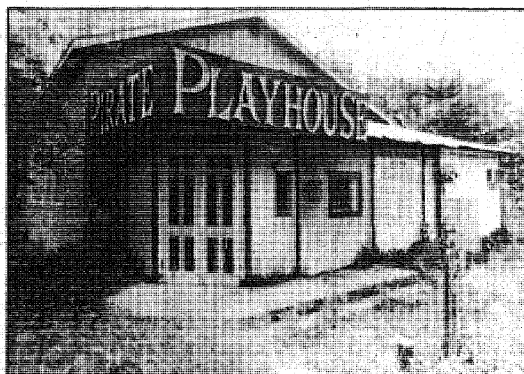
The Pirate Playhouse on Periwinkle Way recently received a new coat of paint as part of preparations for the 1985 season under new ownership. Photo by Mark Johnson.
