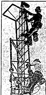
Paul Saha and Kevin Braggaw of Gulf Coast Tower Company install the osprey platform. Photo by David Dugardin.
