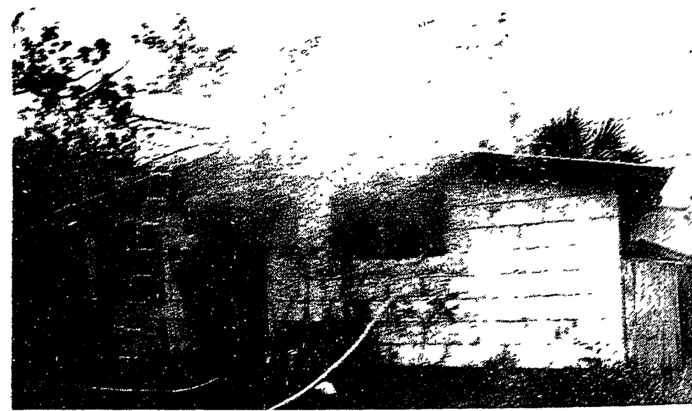
The tenant of this uninjured cottage lost all her belongings in the fire last Wednesday morning.
