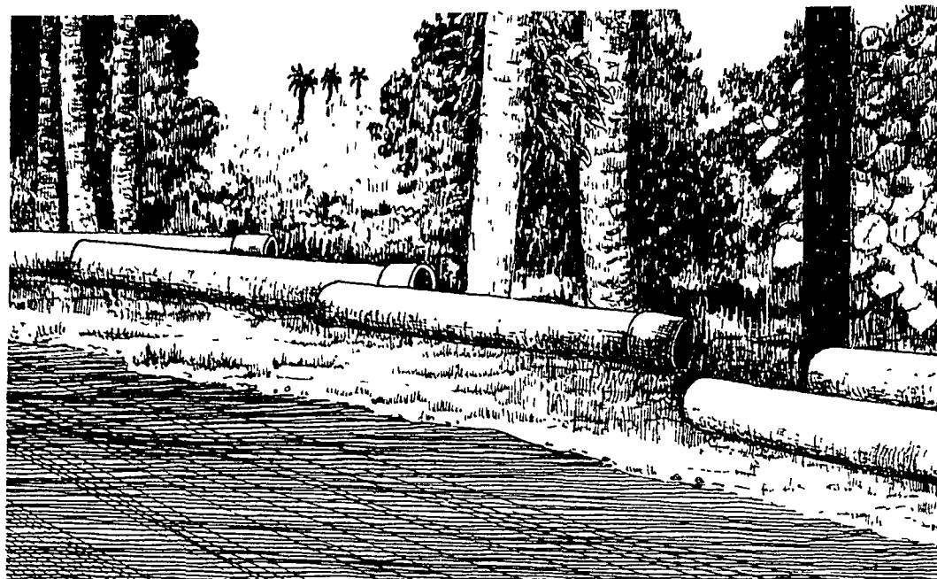
A common sight on Sanibel about a decade ago was a lot of asbestos-cement pipe lying at the side of the road, waiting to be installed underground. Today more than 24 miles of the pipe are buried on the Islands. Out of sight, out of mind.
