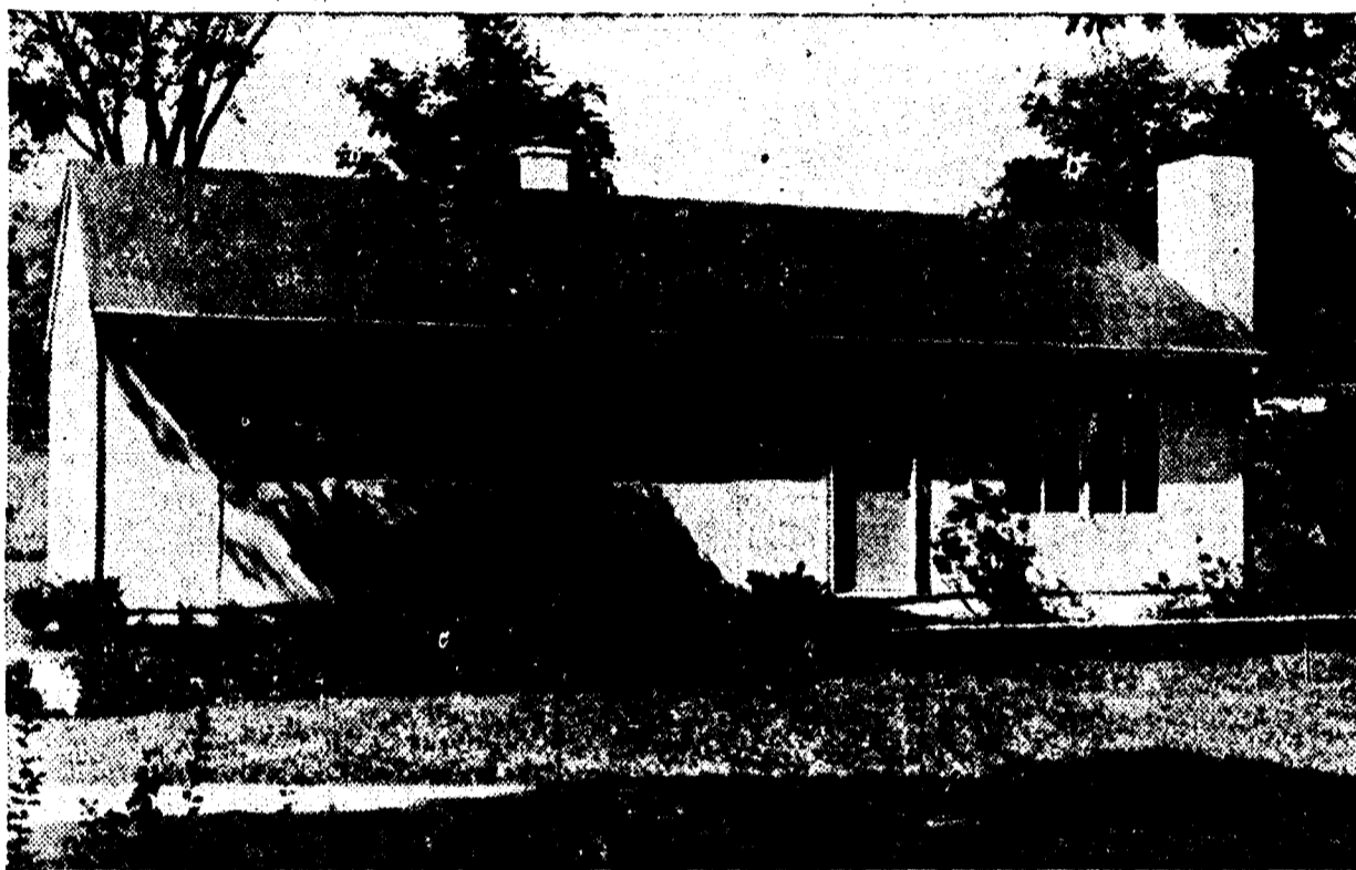
A STEEL FRAME COVERED with steel panels makes the exterior construction of the house, which is shipped in a knocked-down condition and all
