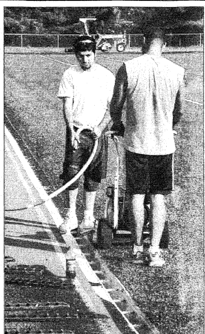
CONVERSION COMPLETE — The conversion of Tatlock Field in Summit from natural to artificial turf was completed this month as crews from Texas-based Sportex finished grooming the completed surface and cleaning the new drainage system, which circles the surrounding track. The Hilltoppers' first home football game on the re-christened Metro Homes Field is scheduled for Saturday, Oct. 8. (Photo by Michael J. Kelly)
