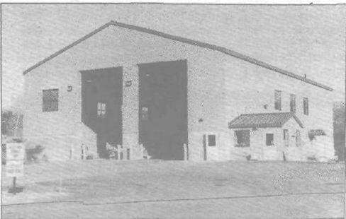
A regional refuse transfer station serving the Central Naugatuck Valley Council of Governments' municipalities opened in Watertown in early December. — Times Photo, Valuckas
