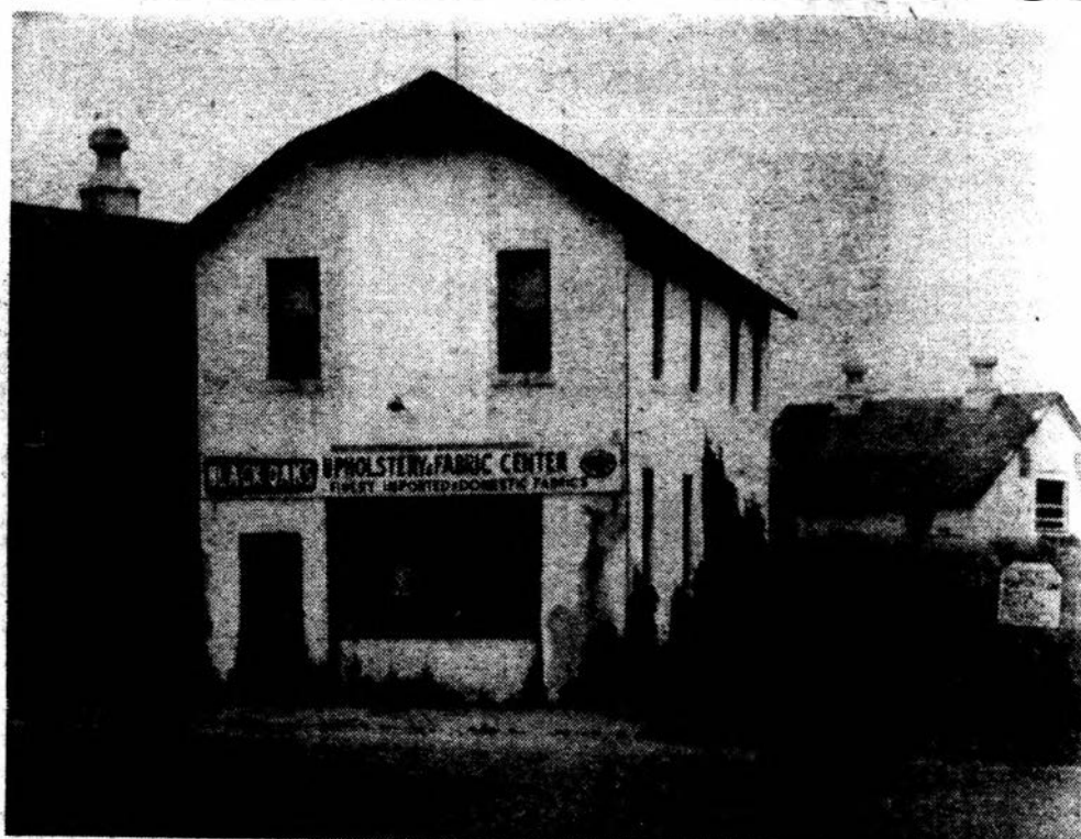
ORIGINAL FIRE HOUSE —This modest looking building was, before 1946, the home of the Pompton Falls Volunteer Fire Company No. 3. One can see where the fire trucks would enter and exit.
